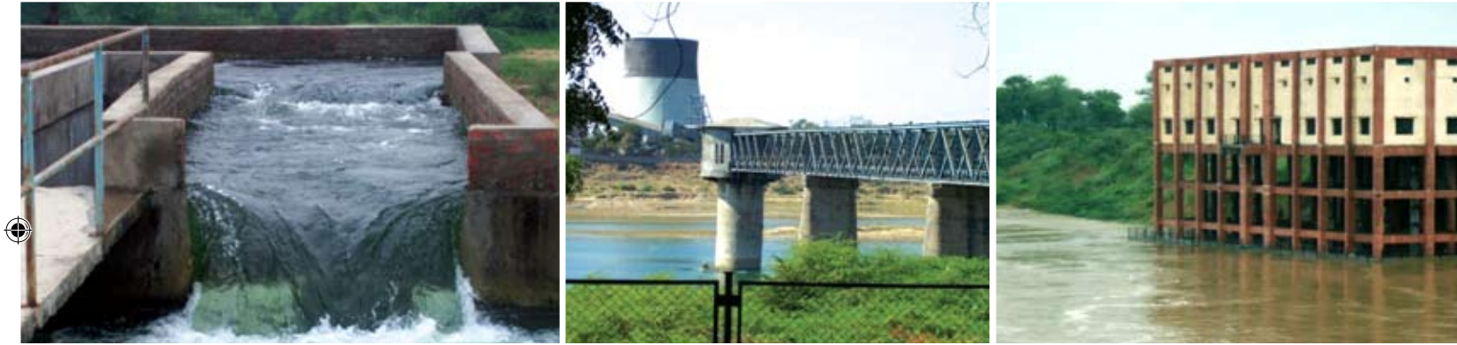
Narmada Canal Raw Water Total Capacity - 350 MLD French Well 07 Nos. Total Capacity - 350 MLD Intake Well I & II Total Capacity - 495 MLD
